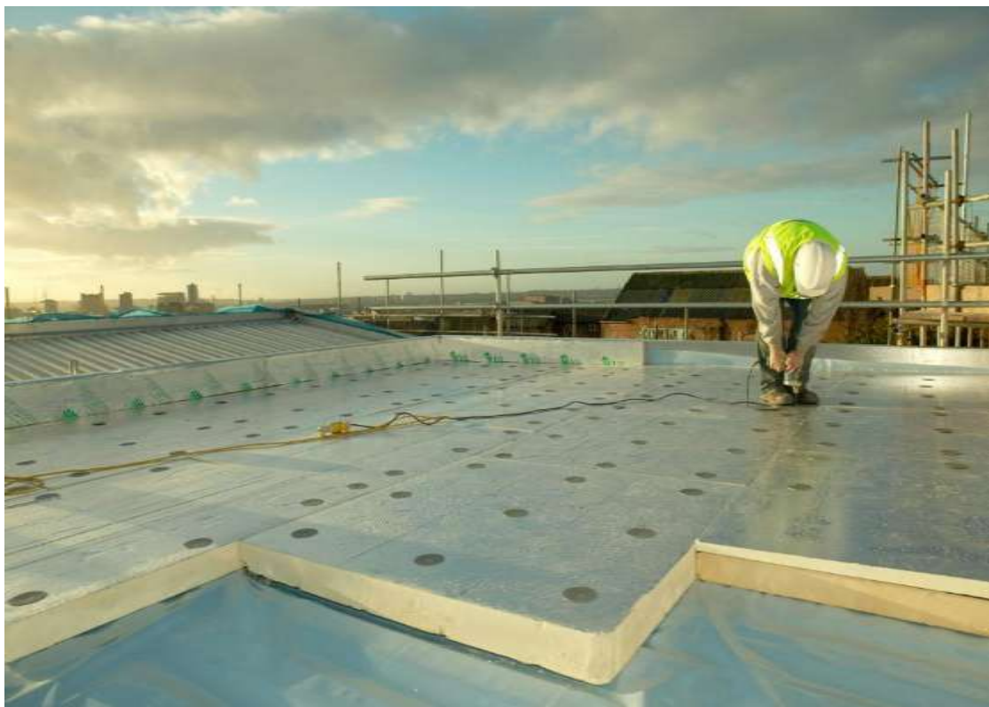
Figure 4.4. Flat roof installation process
