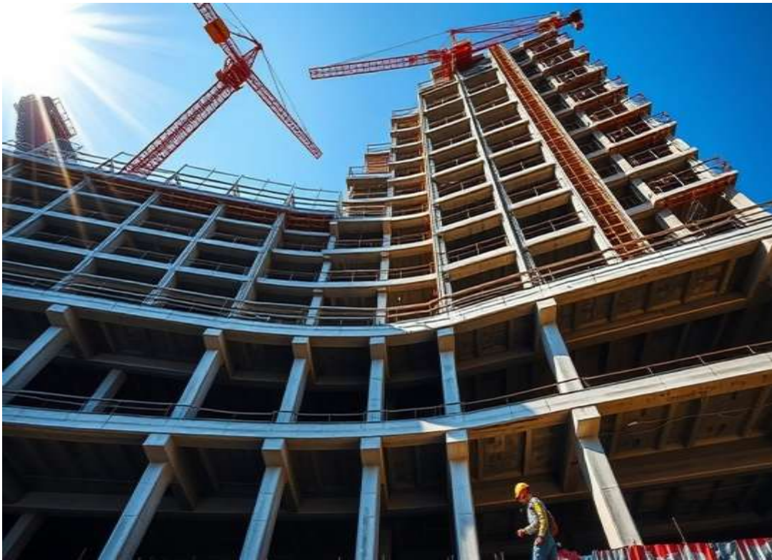
Figure 4.1. Reinforced concrete core
