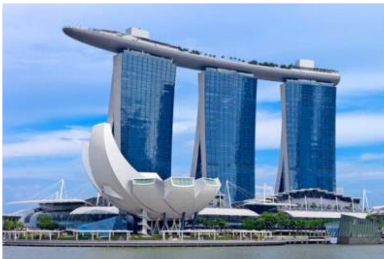
Figure 1.21 – General view of the "Marina Bay Sands" mixed-use complex
