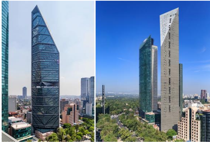
Figure 1.8. General view of the Torre Reforma
