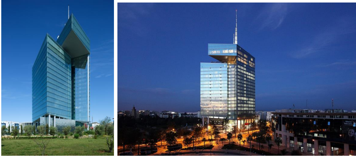
Figure 1.14. General view of the Maroc Telecom HQ
