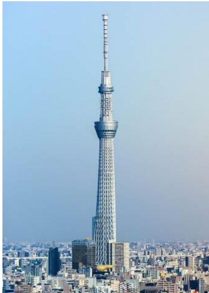
Figure 4.1 – Tokyo Skytree Tower. Tokyo, Japan, the tallest tower in the world. Height 634 m. Year of construction – 2012. Construction – metal.
