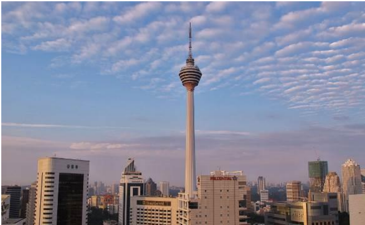
Figure 4.4 – Menara TV Tower in Kuala Lumpur,
