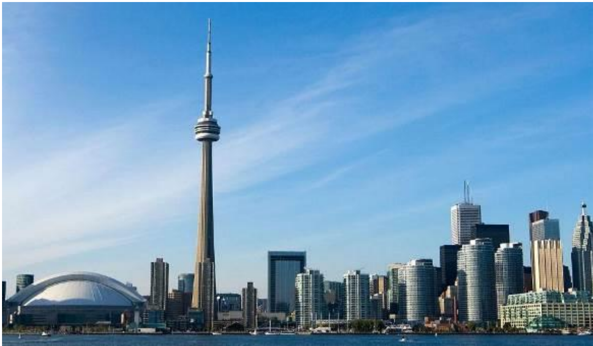
Figure 4.2 – CN Tower, Toronto, Canada, height 554 m, year of construction 1976. Structures – reinforced concrete
