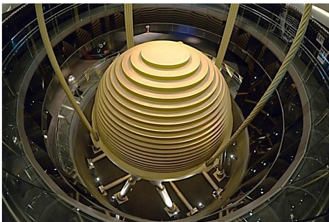
Figure 7.9 – Spherical damper in Taipei 101
